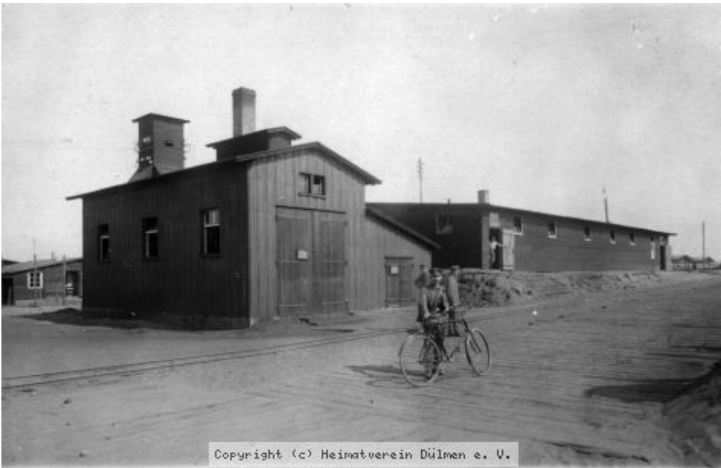
The "Lausoleum", the quarantine and delousing barrack of the camp.
